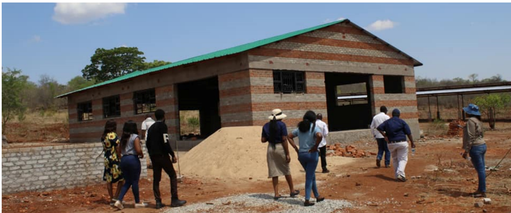
Delegation assessing the abattoir under construction
